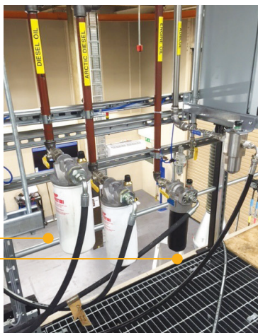
LMP 210 in-line filters and MPS Spin-On for diesel, engine oil, Diesel exhaust fluid
