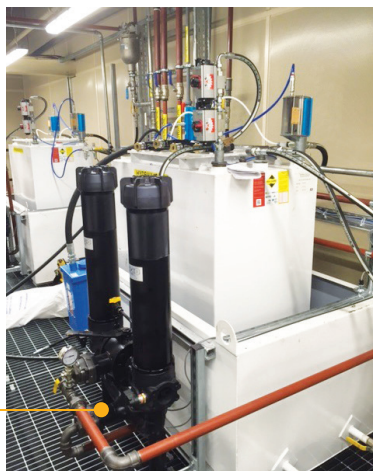
Hydraulic reservoirs with LMD 431 in-line duplex filters
