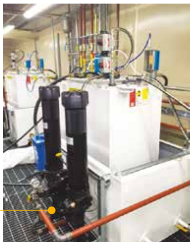
Hydraulic reservoirs with LMD 431 in-line duplex filters
