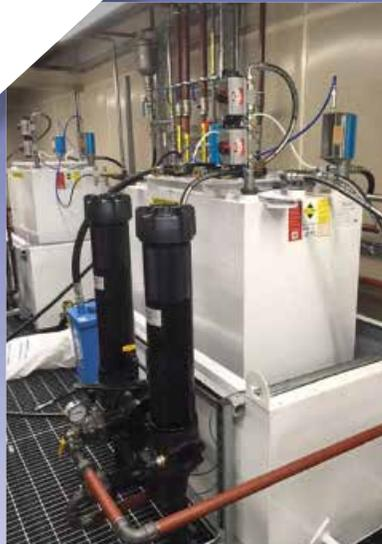
Hydraulic reservoirs with LMD 431 in-line duplex filters
