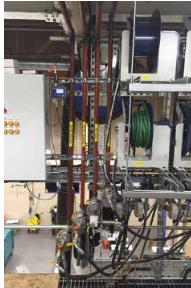
Fluid hose reels with ICM particle counter
