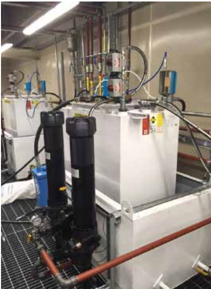
Hydraulic reservoirs with LMD 431 in-line duplex filters
